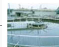
For wastewater treatment
