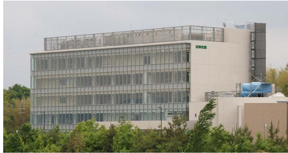
Katsura Research Laboratory under construction
