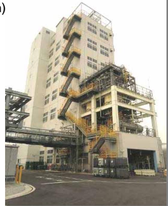
AOA plant at the Kinuura Factory Installing pilot plant
