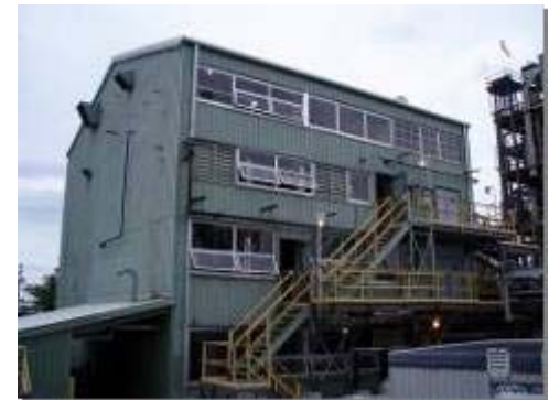
Sanyo Chemical & Resins, LLC
