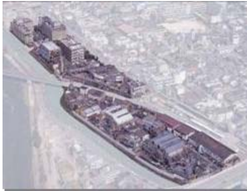
Kyoto Factory, Head Office and Research Laboratory (Higashiyama-ku, Kyoto) Area: approx. 26,000 m 2
