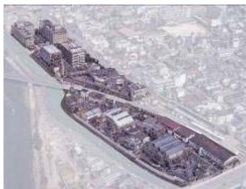
Kyoto Factory, Head Office and Research Laboratory (Higashiyama-ku, Kyoto) Area: approx. 26,000 m 2
