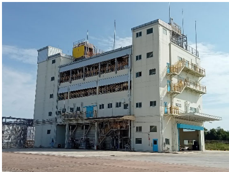
Appearance of the new plant
