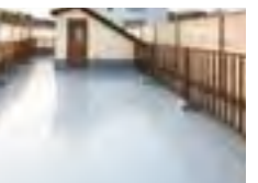
For waterproofing for roofs
