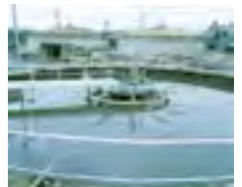
For wastewater treatment
